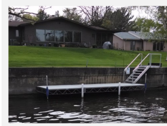
Retaining wall Stair & Dock system
