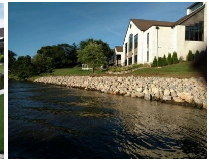
Shore Stabilization with- Limestone Rip Rap wall
